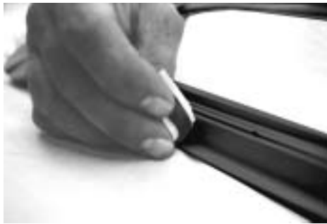
Step 10 - application of butyl to frame
