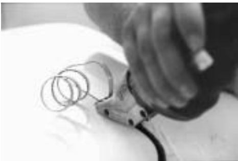
Step 7 - cutting hole in roof panel
