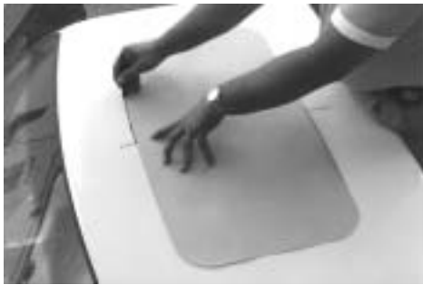
Step 6 - positioning template on roof
